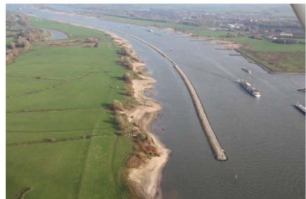
Figure 2. The LTD in the Waal River near Ophemert, looking upstream. Picture from Rijkswaterstaat Oost-Nederland.
